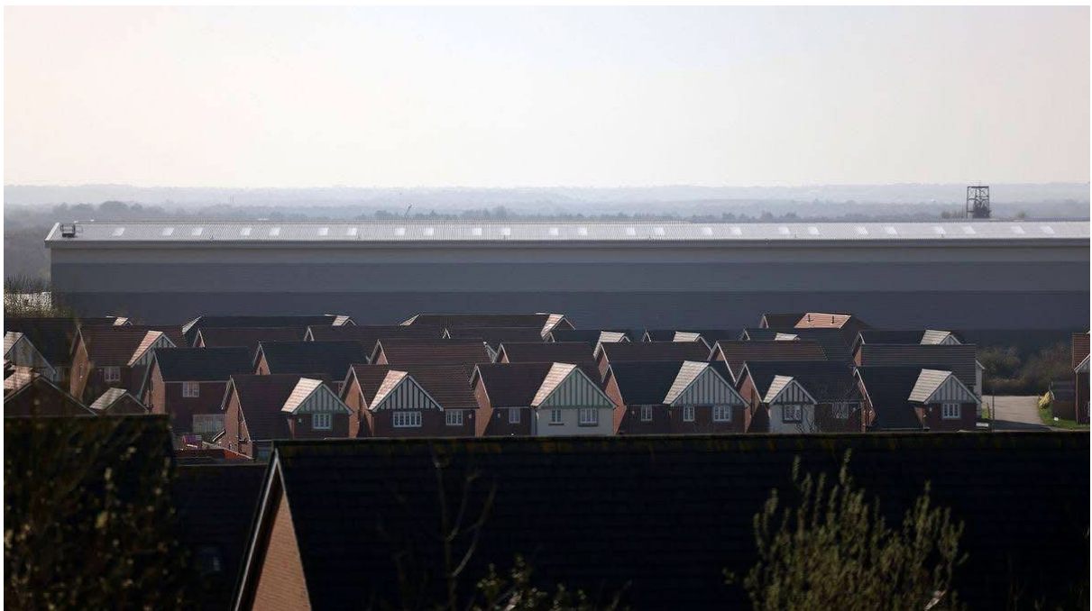
Figure 9: Distant view showing the warehouse roofline extending across the full width of the residential development. Photograph: G Moore, March 2026.
