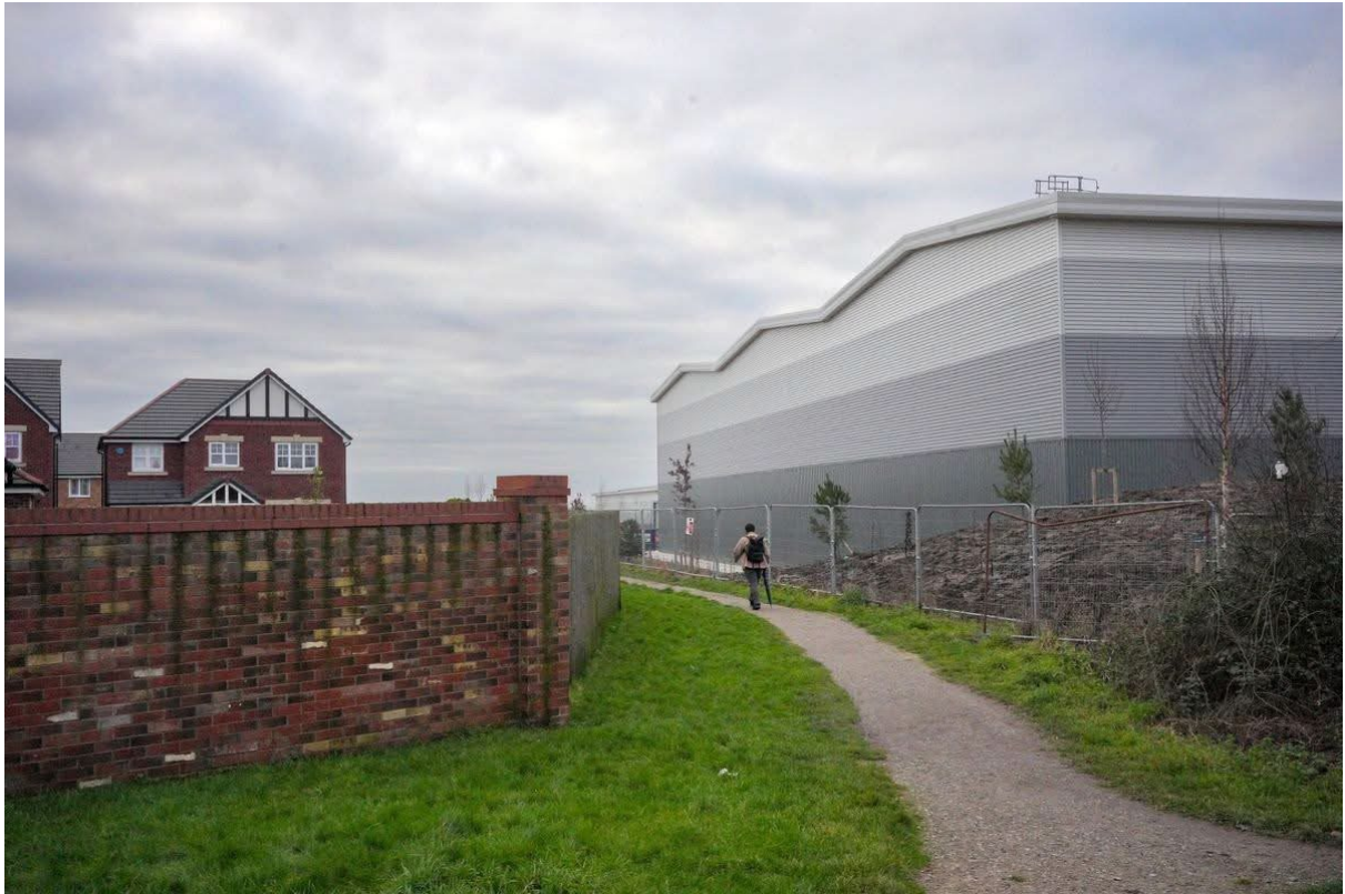
Figure 8: View from a public footpath showing an 18-metre logistics warehouse immediately adjacent to the Henford Estate residential development. Photograph: G Moore, March 2026.
