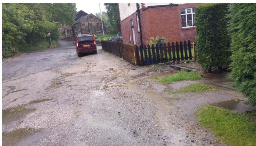
Site Overview and Flooding Impacts
