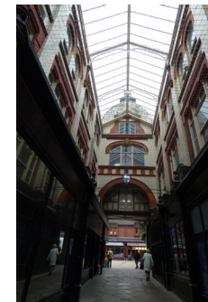
Hilton Arcade, interior rooflight and glazed brick at upper storeys
