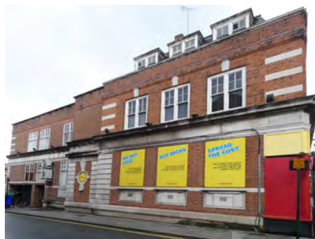
22-24 Yorkshire Street, east return elevation
