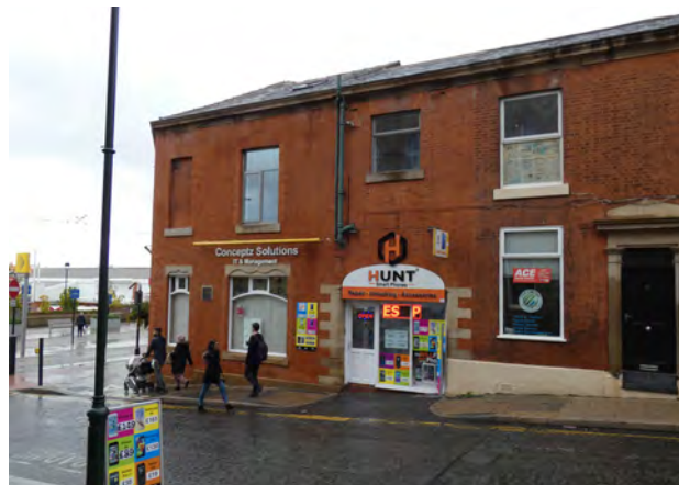
Plate 8.9 Poor shopfront infilling historic archway at southern end of Clegg Street
