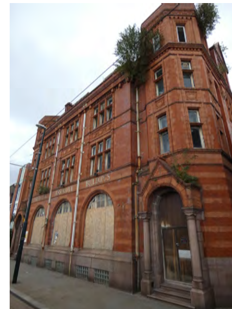
Effective care of vacant buildings is key
