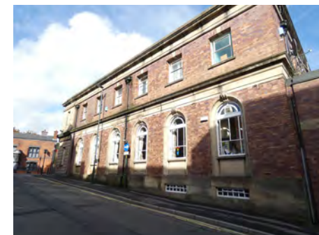
50 Yorkshire Street, east return elevation to Waterloo Street
