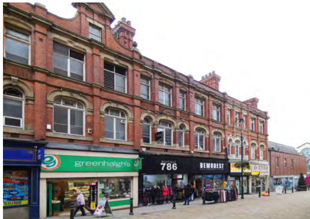
Plate 5.12 Poor retail frontage along Curzon Street at ground floor to Hilton Arcade group
