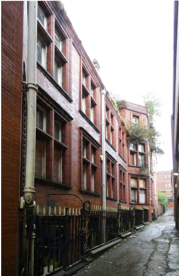
Plate 5.28 Alley running alongside Prudential Building
