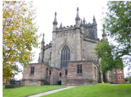
St. Mary's Church, south elevation
