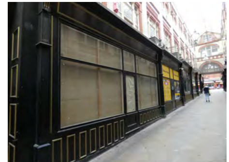
Hilton Arcade, disused shopfront
