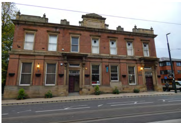
Plate 5.45 Former Post Office
