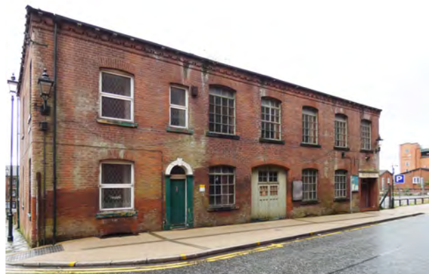
Plate 9.32 1 - 3 Ascroft Street, front elevation
