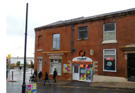
44 Clegg Street & eastern return of 93 Union Street
