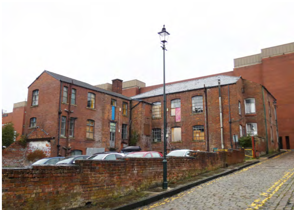
Plate 9.30 Rear elevation of Ascroft Street buildings including historic boundary wall and cobbled roadway to Harrison Street
