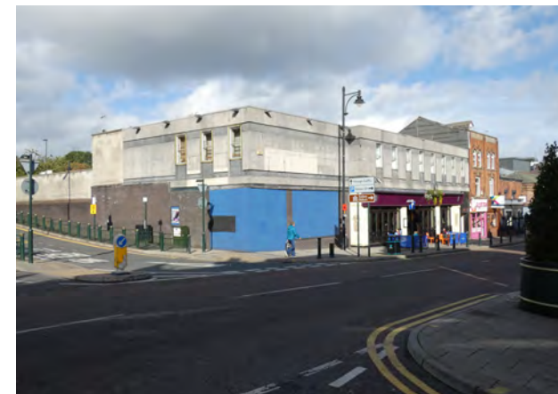
Plate 9.22 Modern block on corner of St Mary's Way and Yorkshire which does not follow the established character of the conservation area
