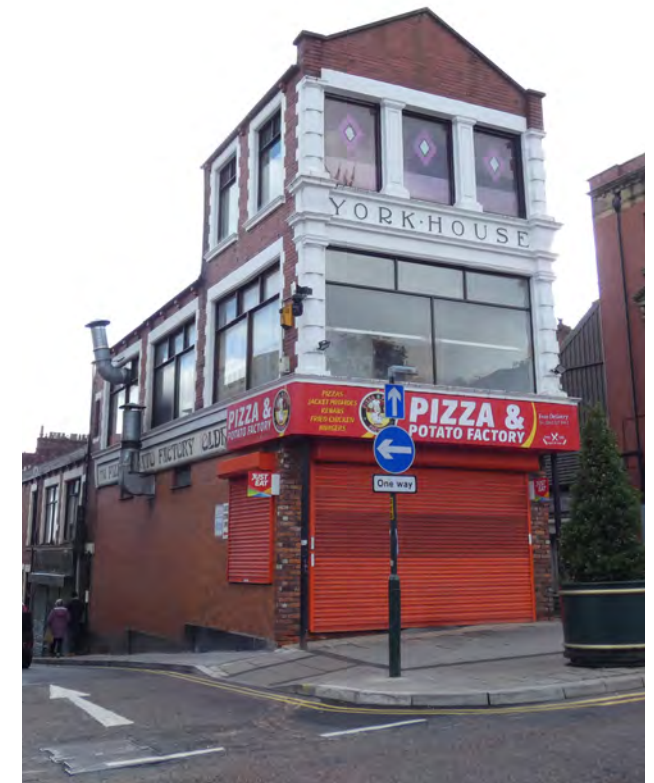
Plate 8.7 32 Yorkshire Street with poor shopfront and signage, roller shutters and unsightly flues
