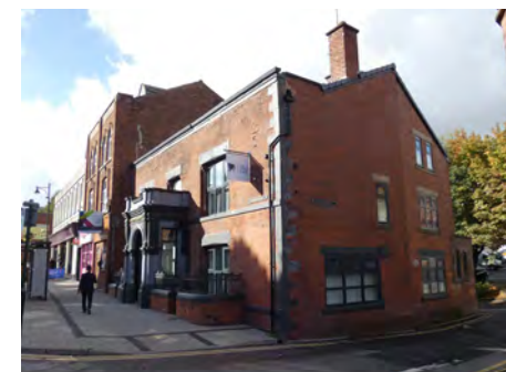
63-65 Yorkshire Street, east return elevation
