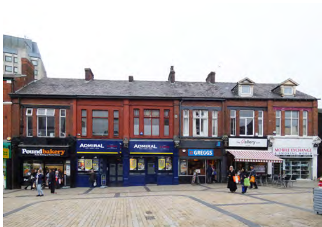
Plate 9.9 19 th century terrace of shops on Henshaw Street
