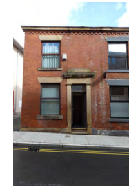
3 Retiro Street, typical range facade
