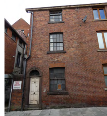
26 Retiro Street, original fenestration
