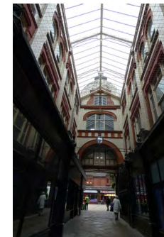
Hilton Arcade, interior roolight and glazed brick at upper storeys
