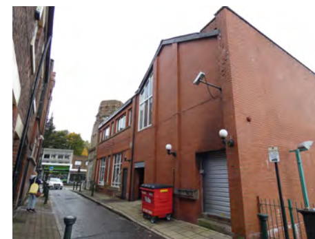
18-20 Yorkshire Street, west return elevation
