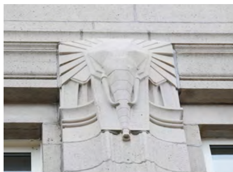
27-31 Market Place, pilaster detail
