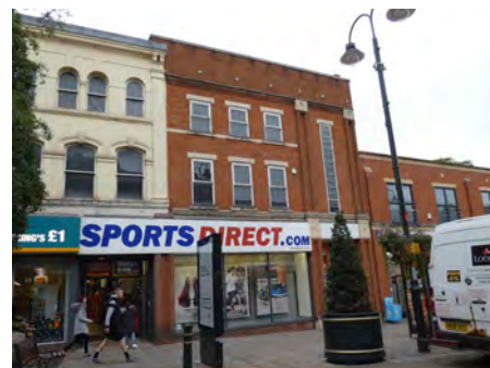
15-17 High Street, east side of frontage
