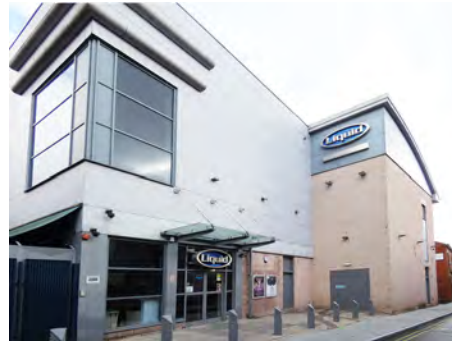
Liquid, Retiro Street
