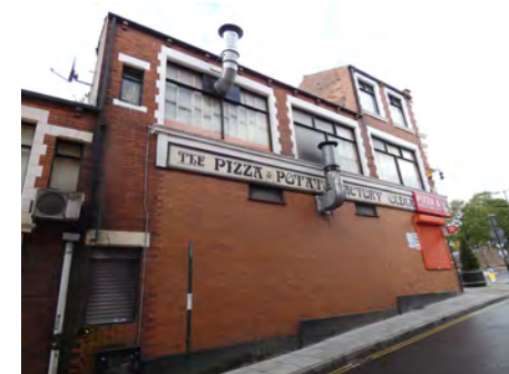
32 Yorkshire Street, east return elevation to Retiro Street
