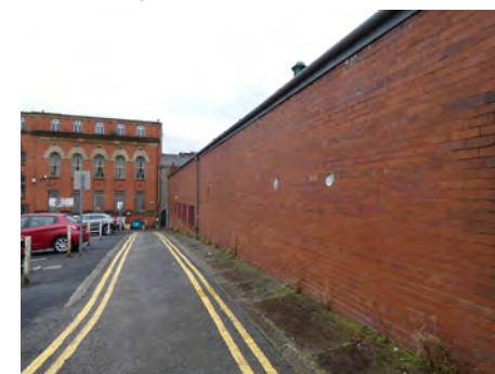
Victoria House, blind rear elevation
