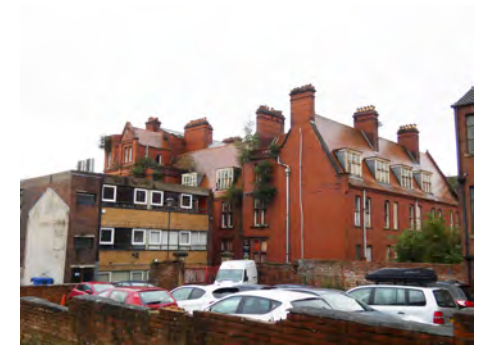
81 Union Street rear elevation, Prudential Assurance Building to west
