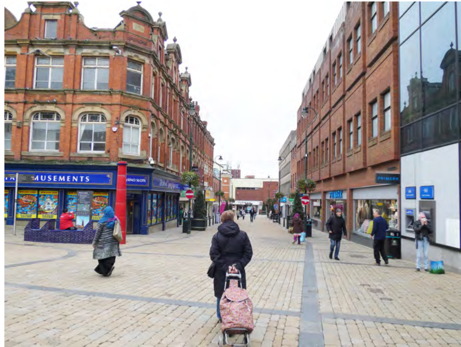
9 Curzon Street, modern facade on right
