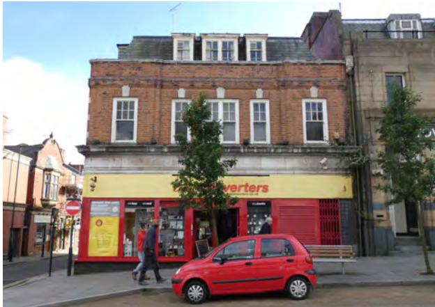
Plate 5.32 Impact of poor quality retail frontage, roller shutters and signage on quality of building above at 22-24 Yorkshire Street
