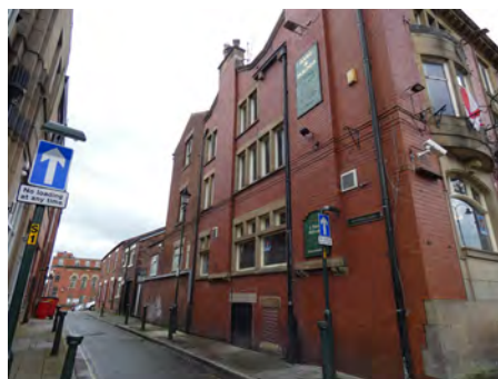
16 Yorkshire Street, east return elevation
