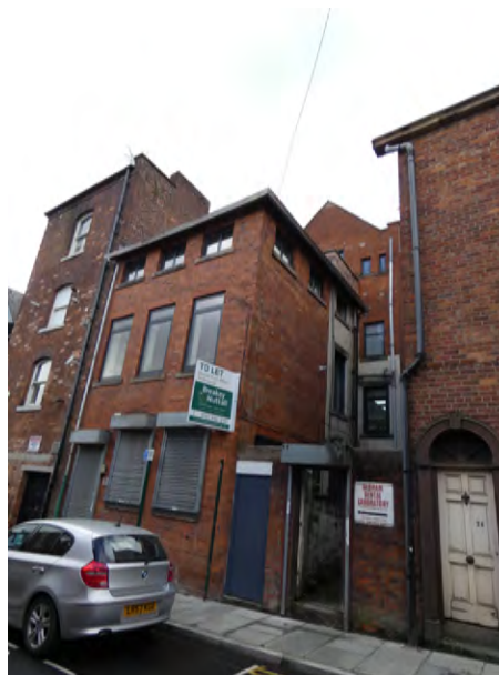
28 Retiro Street, north return elevation
