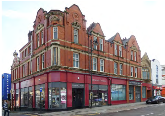
Plate 9.17 Handsome group of late 19 th century buildings at 34 - 48 Yorkshire Street which make a positive contribution to the conservation area
