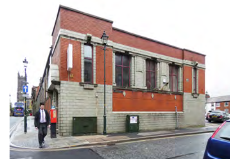
Victoria House, south elevation to Firth Street
