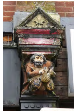
Plate 9.11 Carved capital and corbel brackets to 19 th century retail frontage on Henshaw Street
