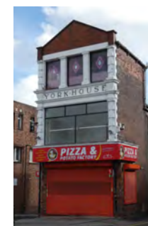
32 Yorkshire Street and east return elevation to Plate Street
