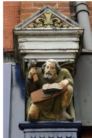
Plate 9.10 Carved capital and corbel brackets to 19 th century retail frontage on Henshaw Street
