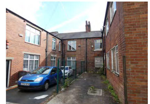
113 Union Street, rear closet wings with no. 115
