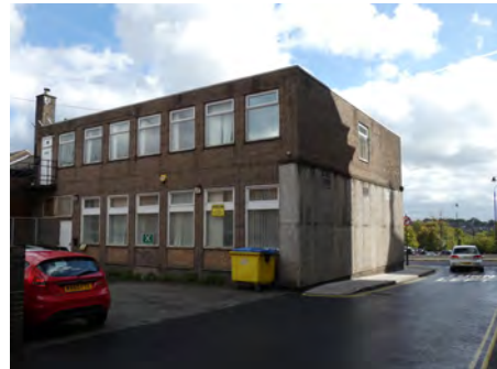
111 Union Street, rear elevation to Walter Street
