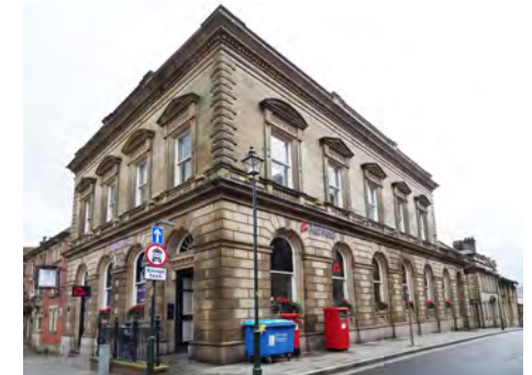
10 Yorkshire Street, west return elevation
