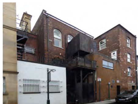
31 Queen Street, rear elevation
