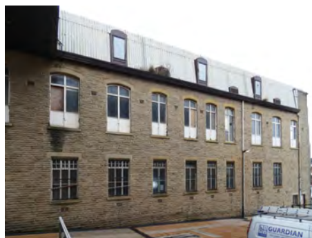
88 Union Street, Oldham Library rear elevation
