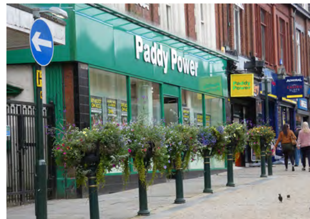
Plate 9.15 Poor signage and shopfronts within proposed extension
