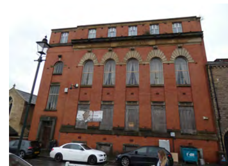
105 Union Street, rear elevation to Firth Street
