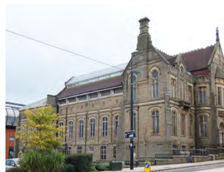
88 Union Street, Oldham Library east elevation
