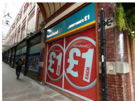
15 High Street, detracting shopfront to Hilton Arcade
