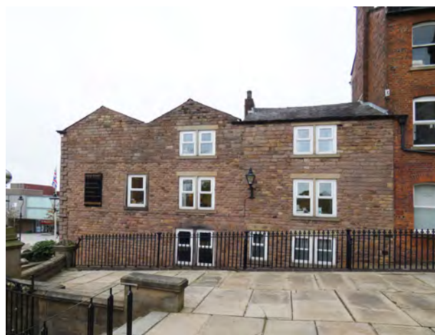
Plate 5.52 11 Church Terrace side return to Church Passage with sandstone finish
