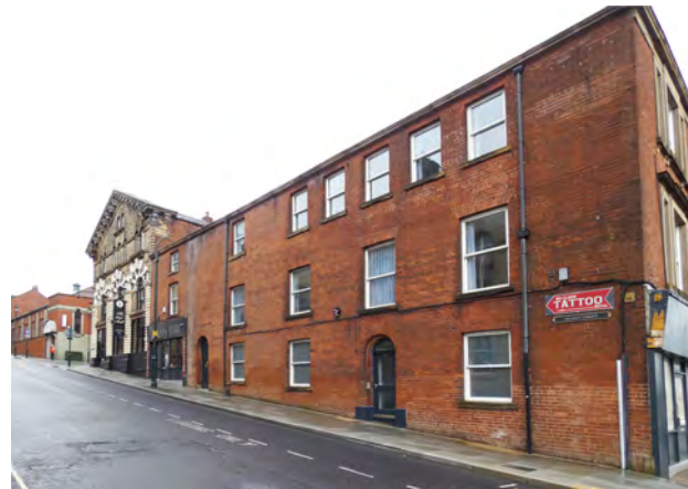
Plate 5.24 Looking north along Greaves Street and run of high quality buildings which mediate change in levels and form worthy neighbours to listed Town Hall
