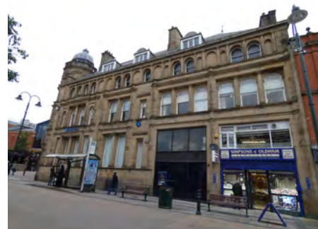
25-37 High Street, principal south elevation
