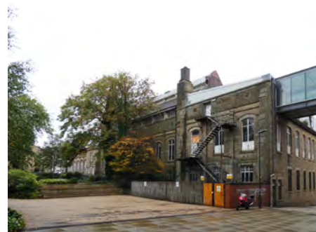
88 Union Street, Oldham Library west elevation
