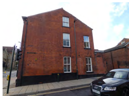
117 Union Street, east return elevation to Waterloo Street
