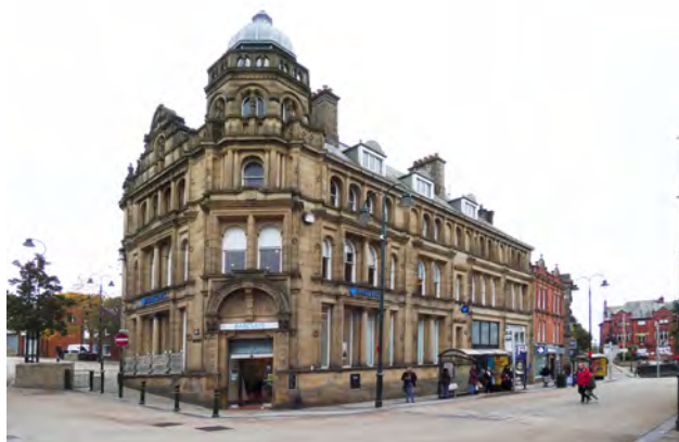
Plate 5.13 Grade II-listed Barclays Bank on the corner with Church Terrace and the Greaves Arms positioned behind
