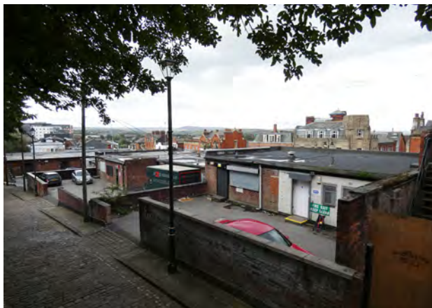
Plate 9.21 Rear side of 21 - 41 Yorkshire Street block providing poor backdrop to the historic character of Church Street
