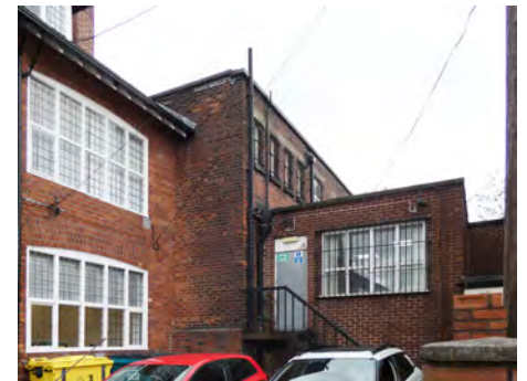
3 Greaves Street, rear extension
