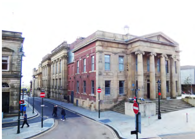
Plate 5.20 Eastern facade of former Town Hall extending southwards along Greaves Street
