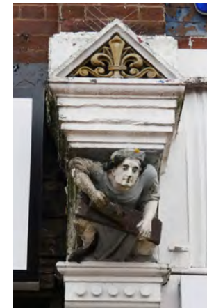
Plate 9.12 Carved capital and corbel brackets to 19 th century retail frontage on Henshaw Street
