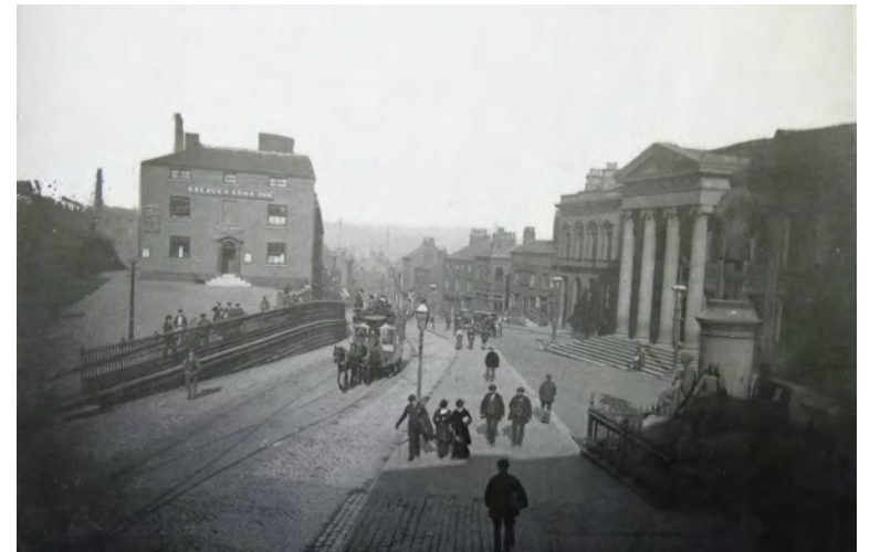
Plate 4.12 Town Hall Square looking east, c. 1900 (Oldham Local Studies & Archives)
