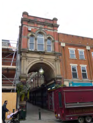
Plate 5.53 South face of Hilton Arcade
