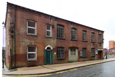
1-3 Ascroft Street, no. 1 to left
