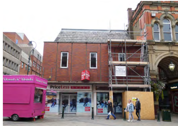
Plate 8.1 1-3 High Street detracting from the composition, scale and detailing of the Hilton Arcade block
