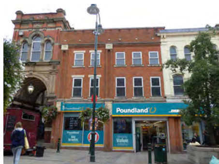
15-17 High Street, west side of frontage
