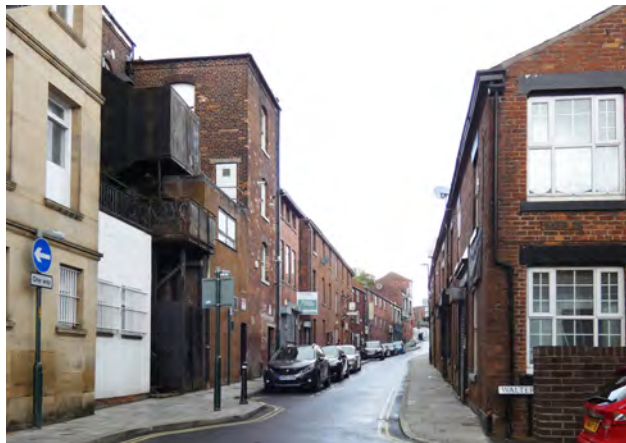
Plate 5.23 Looking north along Retiro Street, only left side is currently within conservation area
