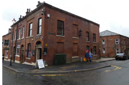
22 Clegg Street, north elevation to Ascroft Street
