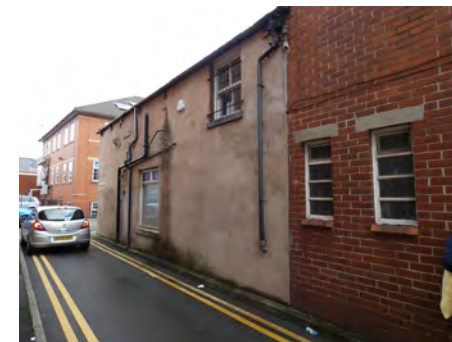
18 Waterloo Street, return north elevation
