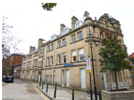
25-37 High Street, north elevation to Church Lane
