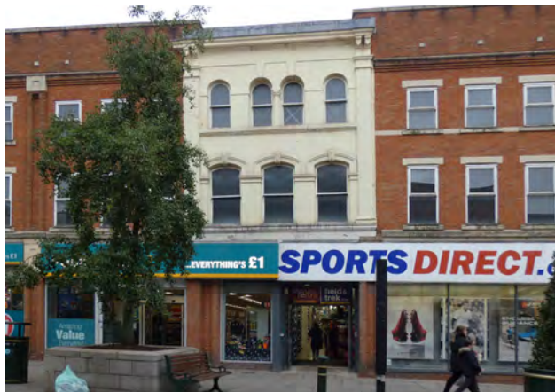
Plate 8.8 Poor shopfronts and signage across 15 -17 High Street which fails to relate to architecture of building above
