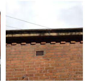
3-21 Retiro Street, dentil detail
