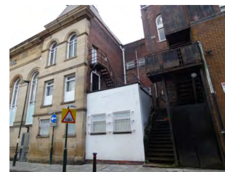
109 Union Street, east elevation to Retiro Street
