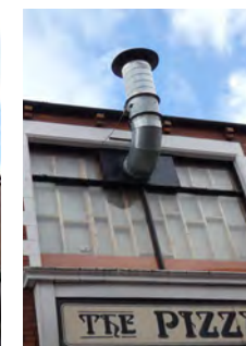
32 Yorkshire Street, visible stud wall and extract services to Retiro Street
