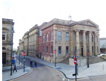
Town Hall and east return to Greaves Street
