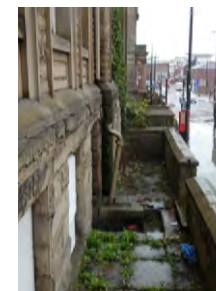
105 Union Street, Masonic Hall lightwell
