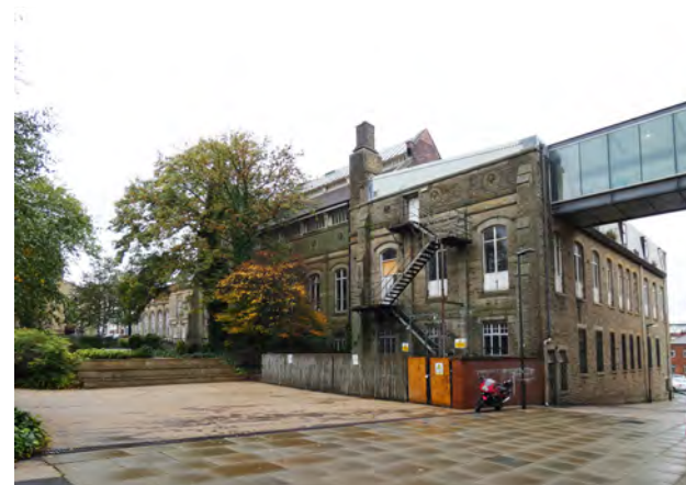
Plate 9.29 Pedestrianised public realm to south side of Cultural Quarter
