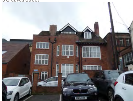
5 Greaves Street, rear elevation
