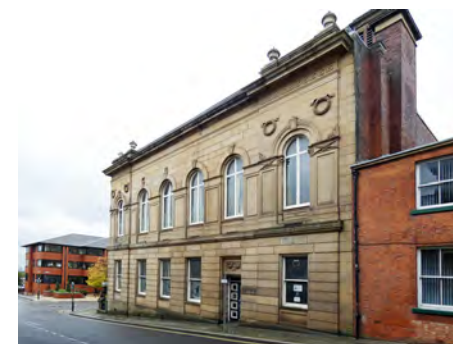
95 Union Street, east elevation to Greaves Street
