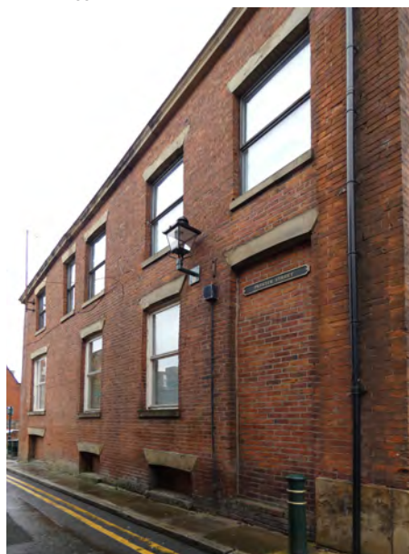
36 Clegg Street, south elevation to Printer Street
