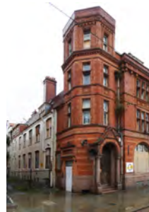
79 Union Street, southwest turret & west elevation
