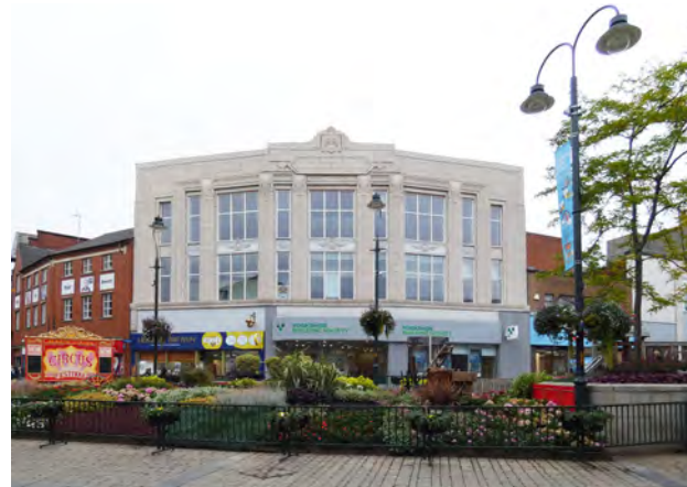
Plate 9.7 Art Deco building turning the corner between Market Place and Henshaw Street with large planted bed in front
