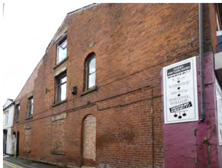
16 Waterloo Street, south return elevation
