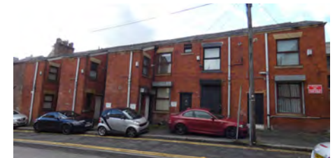
3-21 Retiro Street, rear closet wings
