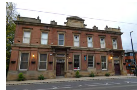
84 Union Street, former Post & Telegraph Office
