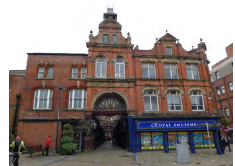
Hilton Arcade, north elevation to Albion Street
