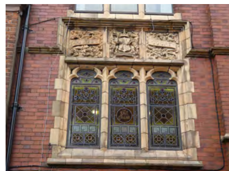
11a Church Lane, first floor window detail
