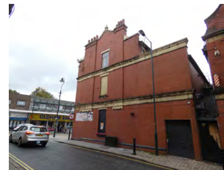
26 Yorkshire Street, west return elevation
