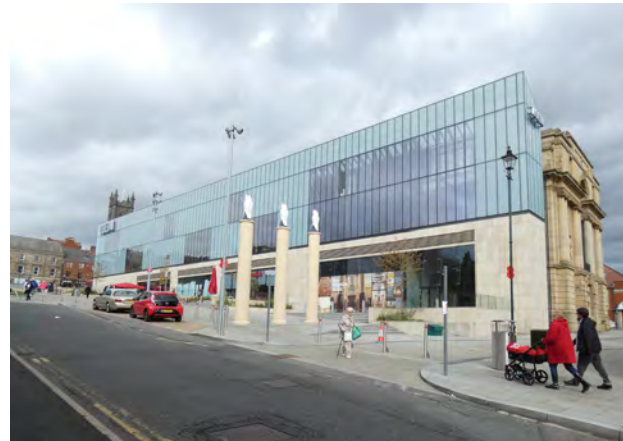
Plate 5.36 Extension to former Town Hall to house new cinema
