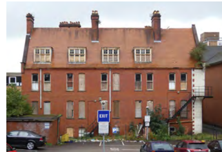
79 Union Street, rear elevation
