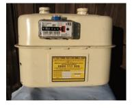
Readings are usually in the form of a numerical value on the box, ignore any digits that appear in red. Readings may also be in the form of a dial and numbers should simply be read in set order.
