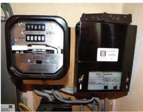
Some meters have two sets of numbers, while others have one, which is the 'day rate'. You may have to press a button to display the 'night rate'.
