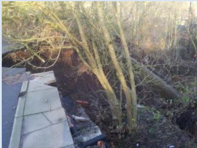
Picture 7 Highway embankment collapse
