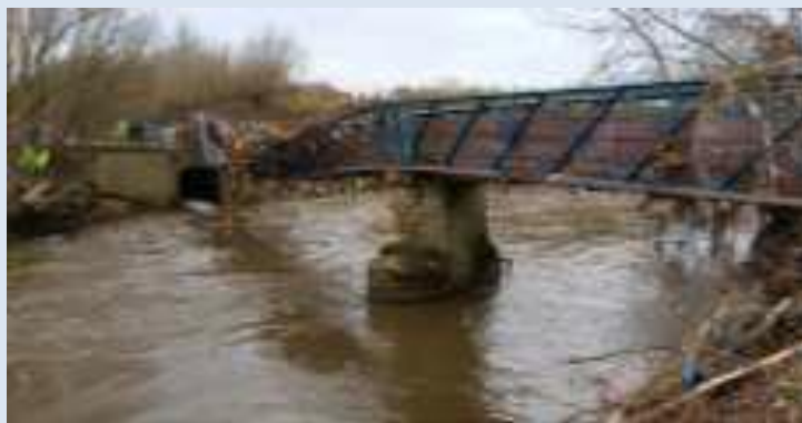
Picture 16 Milltown Street footbridge damaged beyond repair
