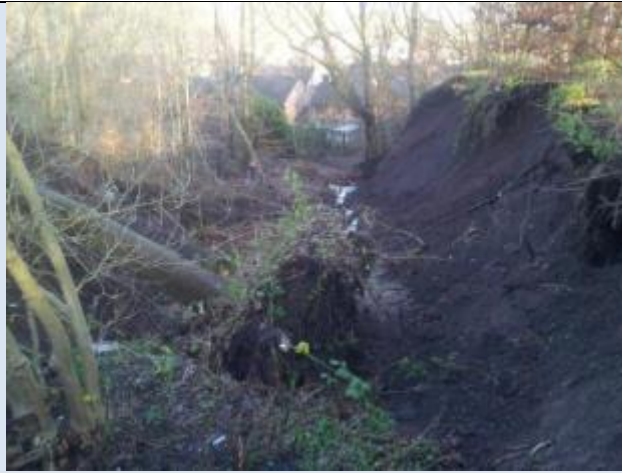
Picture 8 Land Slip showing land eroded by culvert collapse
