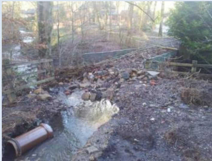
Picture 6 Landslip debris and damage to footbridge
