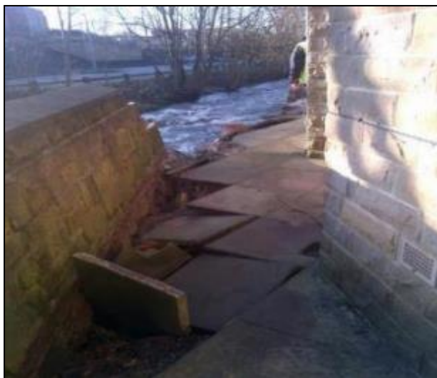
Picture 3 Collapsed section of flood wall at Littleborough
