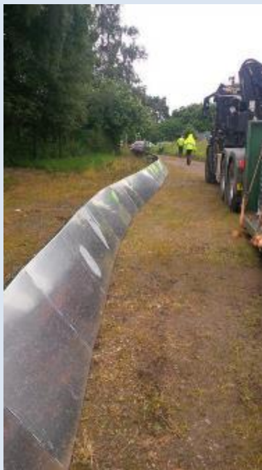
Picture 91 Installation of temporary defences being tested during an exercise in July 2016. These defences aim to improve protection to properties including those which flooded on Boxing Day.
