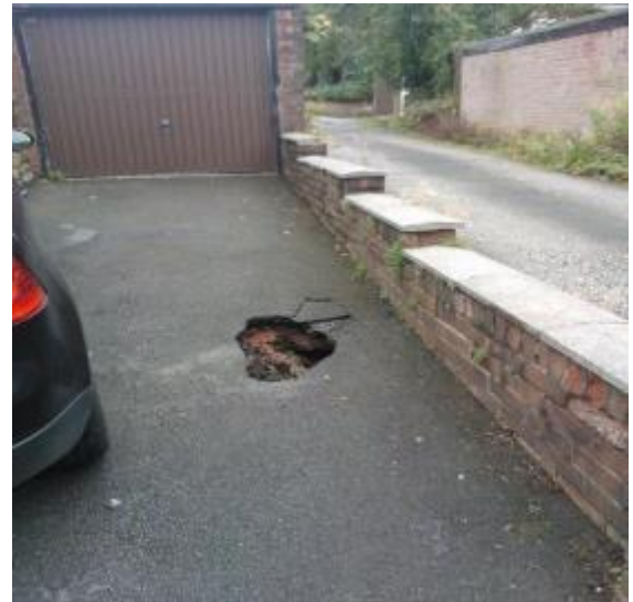
Picture 2 Hole appeared due to Pickhill Brook culvert collapse below
