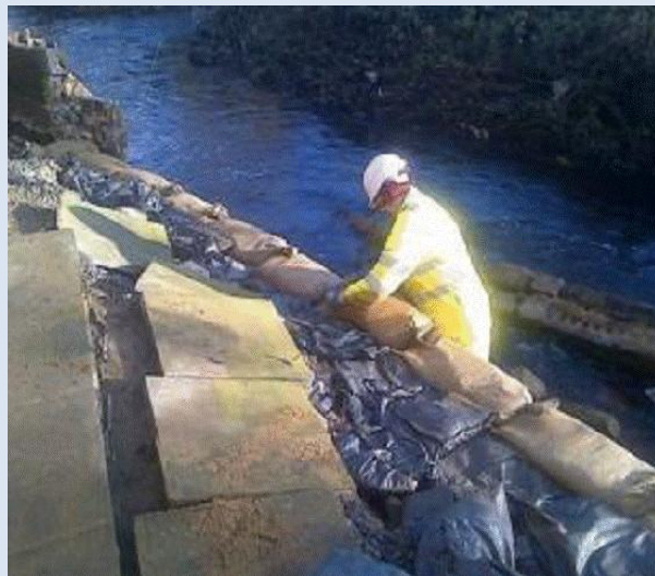
Picture 62 Littleborough Flood Wall Temporary Sandbagging
