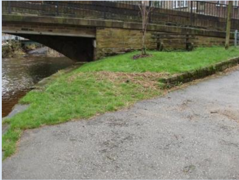
Picture 35 Debris showing the extent of the water that came out of channel at the location of the bridge on High Street, Delph
