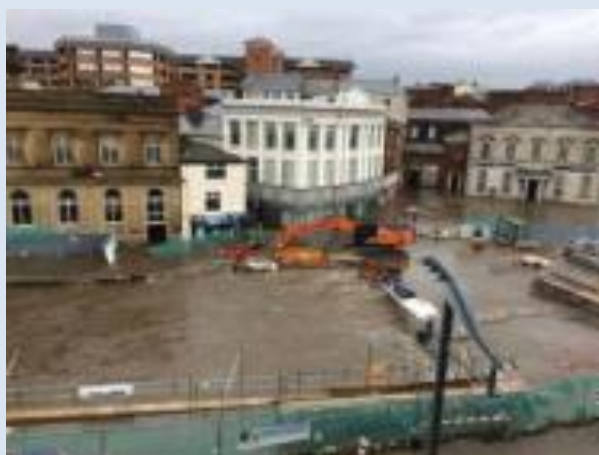
Picture 66 Water re-enters river where culvert is being opened up
