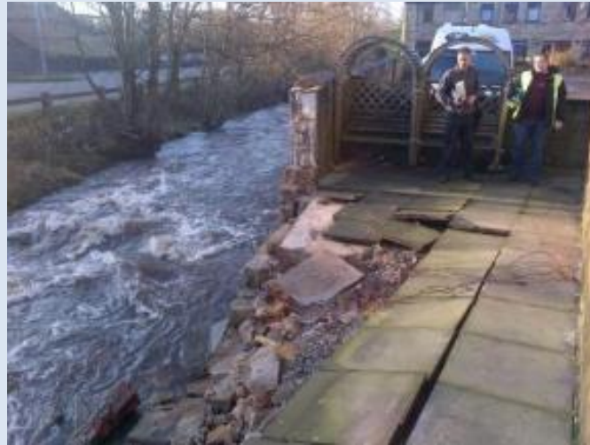
Picture 61 Riverside Nursing Home Flood Wall Collapse
