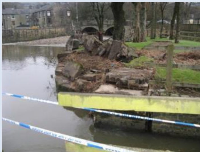
Picture 22 Damage to canoe by-pass of Bridge Street weir
