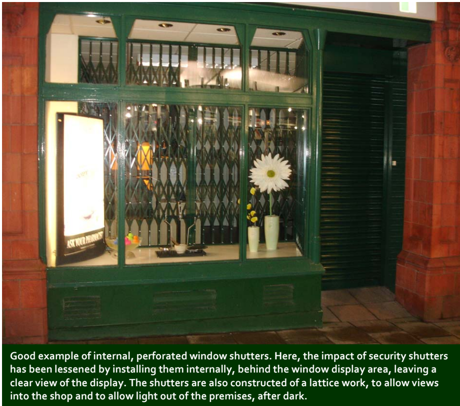
Figure 19 Good example of good internal shutters
