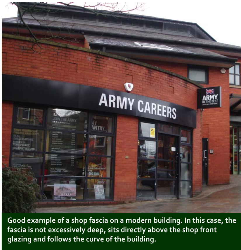
Figure 10 Good example of a modern fascia
