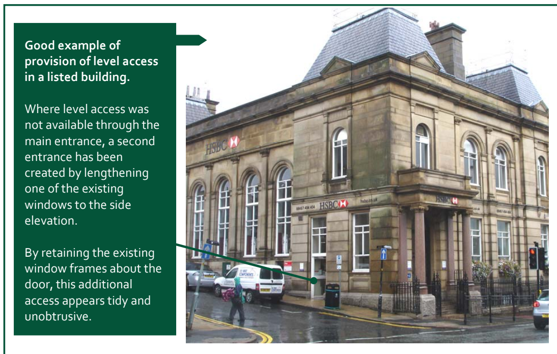
Figure 8 Good example of provision of level access in a listed building
