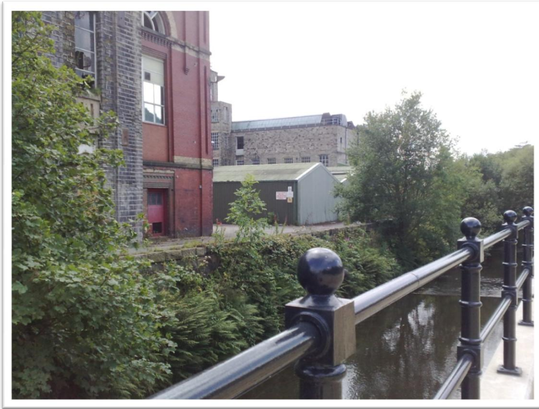
Figure 2-1: Raised Defence at Frenches Wharf, River Tame
