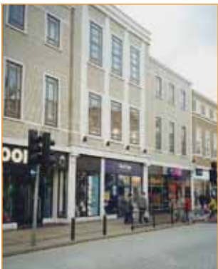
In Wimbledon, a cinema is provided above shops and cafes, so that the 'blank box' is located at the upper floor level not the street
