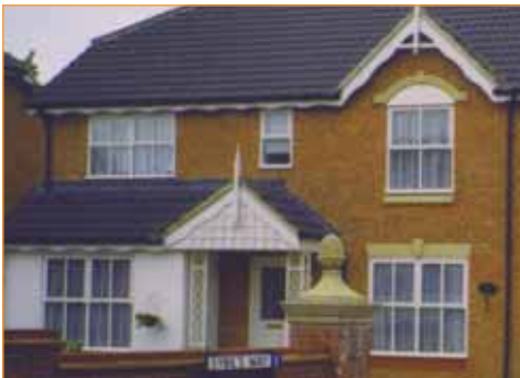
In contrast, this house relies on dormers, barge boards and window details for interest. The poor quality of these details does not create an interesting building.
