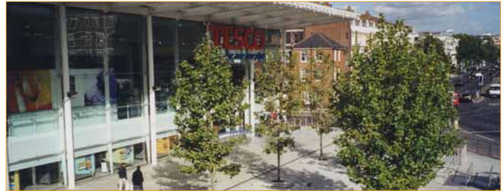
Large supermarket designed to relate positively to the new public open space onto which it fronts
