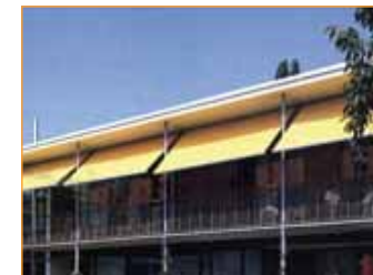
Sun protection allows the use of large glazed areas without the detrimental effect of overheating
