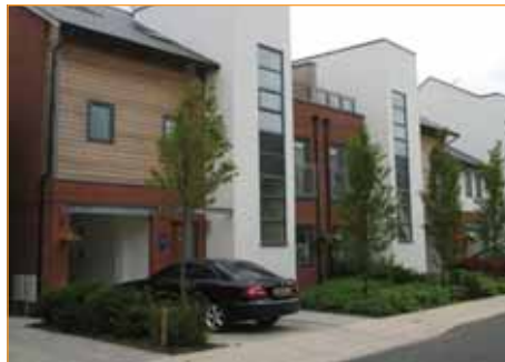
Landscape treatment reduces the impact of on-curtilage car parking on the street-scene
