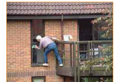
Think about how buildings will be cleaned, so that they can be maintained easily and safely
