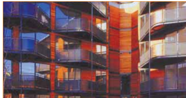
Left: The use of pre-fabricated elements can help to speed up construction as well as ensuring consistent quality
