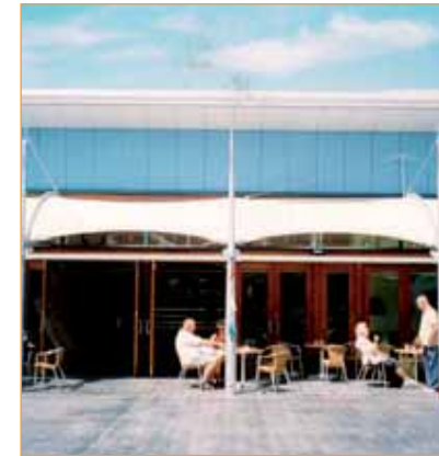
Consistent treatment of shopfronts can enhance a distinctive character of a street
