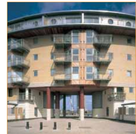
Higher floor-to-ceiling heights on the ground floor allow use as either residential, shops or offices
