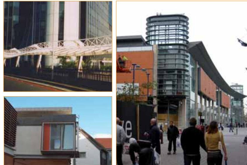
Landmarks and focal points can be of varying character, a special structure, a corner building or a special building element
