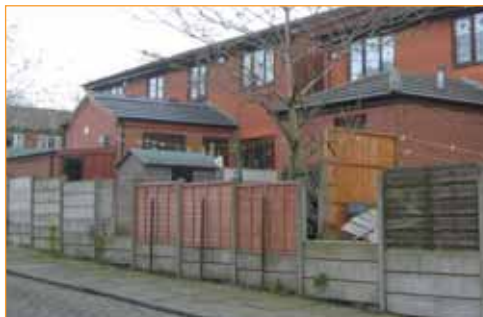
Back along public streets invite vandalism and create a poor street scene
