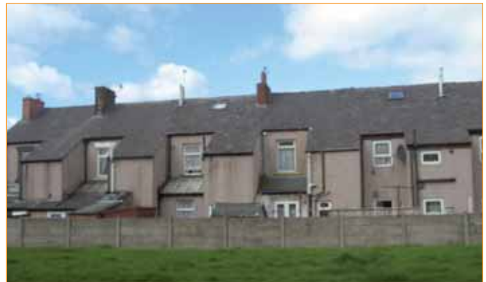
Rear boundaries onto public space are vulnerable to criminals, and are an unattractive edge to the space or street.
