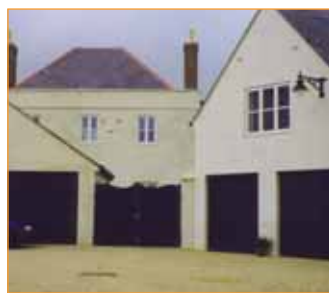
A much less successful courtyard: overlooking is minimal and series of garage doors and gates is forbidding.
