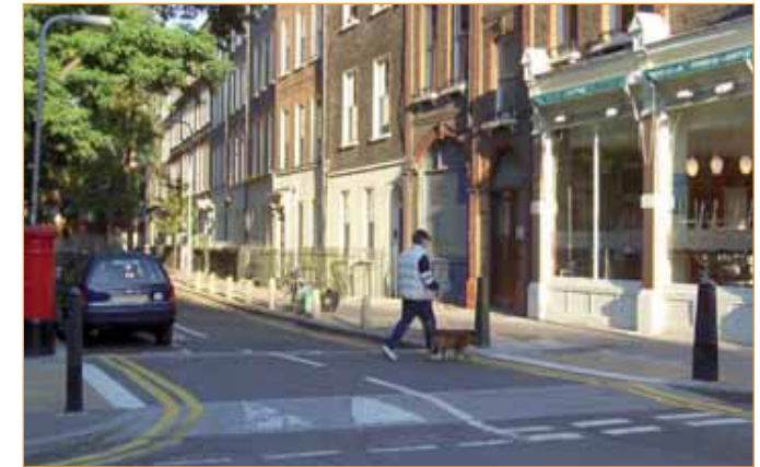
Raised crossings for pedestrians where side roads meet the arterial road make it easier for people to walk along the major road. These 'entry treatments' also help to define changes in character from the main street to the side streets.
