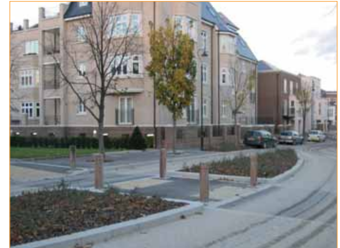
This traffic island makes cars change direction, as well as defining an important pedestrian link to an open space.
