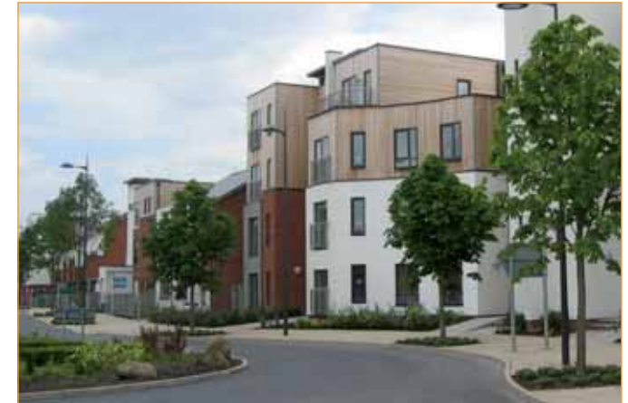
This housing development in Didsbury creates attractive streets that are not just for cars.
