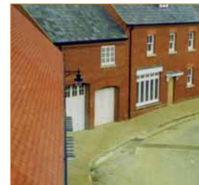
These garages have been designed to appear as workshops or outbuildings, and contribute positively to the street.
