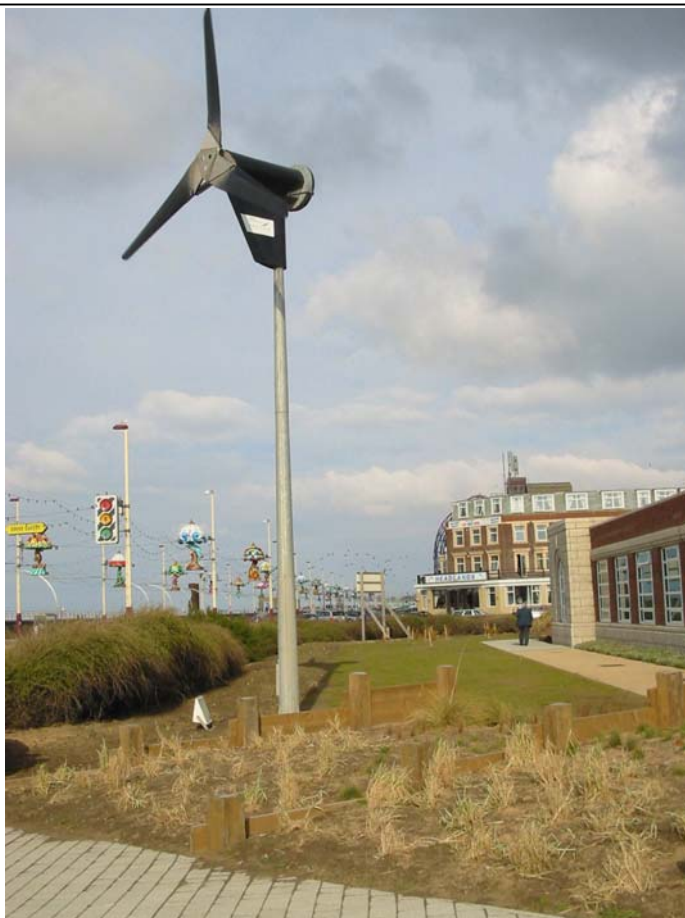
Photo 5. A 6kWh stand alone grid connected 'Proven' wind turbine (hub height 9metres) Blackpool promenade- (Source OMBC)
