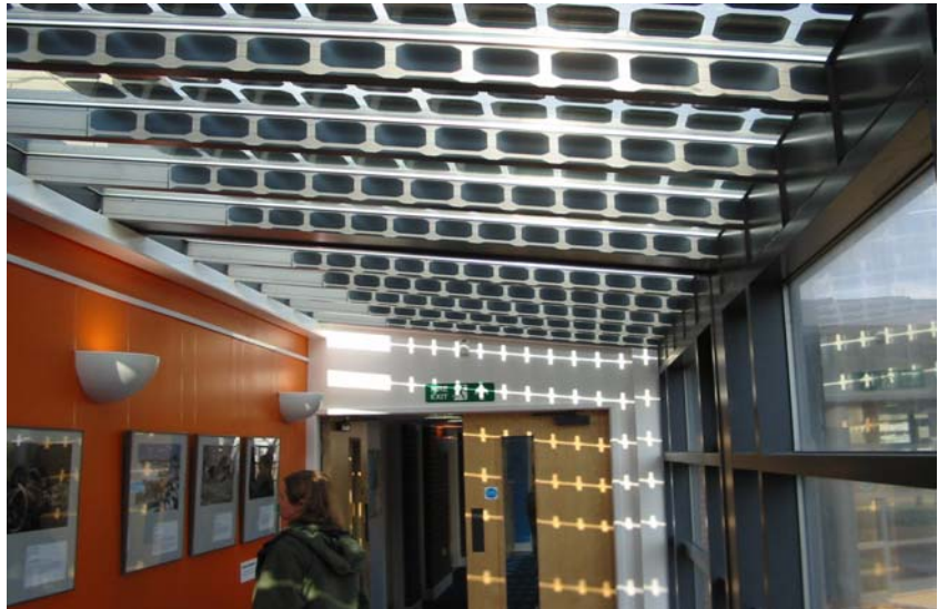
Photo 3. Solar PV panels integrated into glass roofing to provide shading on a converted and refurbished 'Solaris Centre' in Blackpool. Source - OMBC)
